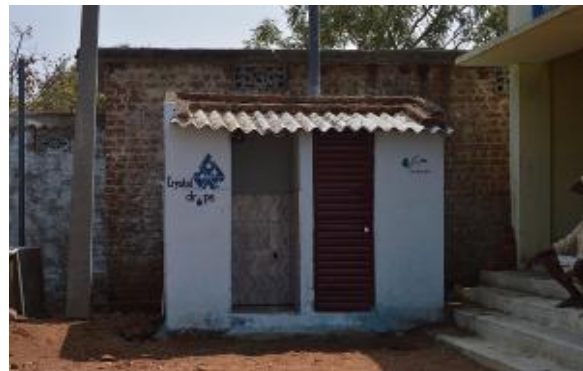
Right: Installed Standard Toilet with added bathroom block 2017
