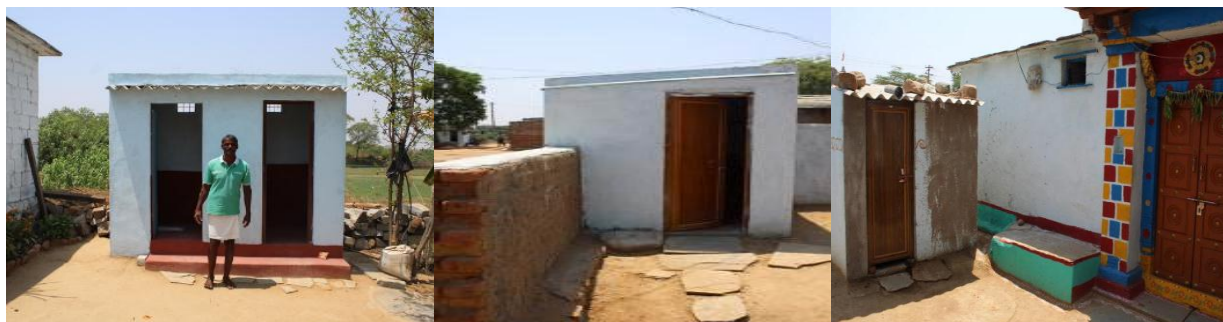
Newly installed IHHL's under Crystal Drops – 2017
