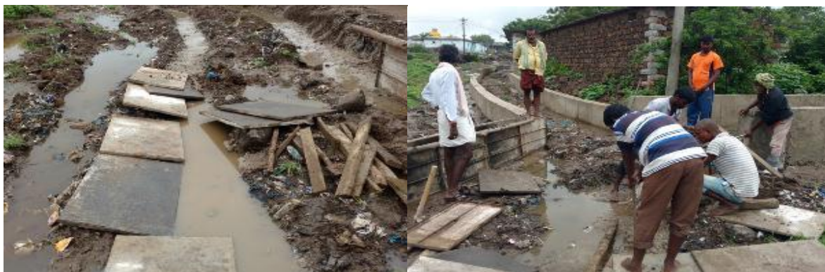
Construction of drainage in Naskal - 2016
