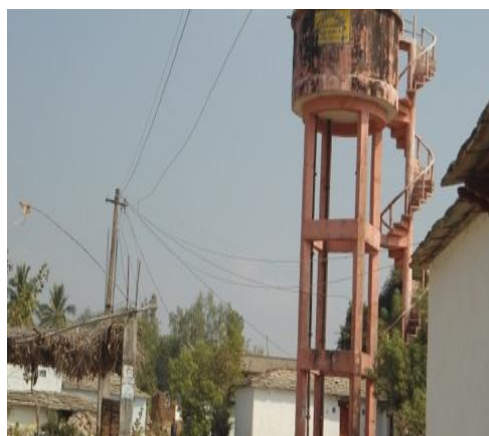
Overhead Service Reservoir located in the village – 2013
