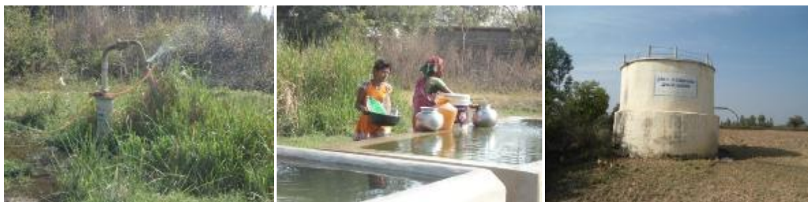
Photographs of the existing Drinking Water Sources in Govindapur Thanda - 2013.
