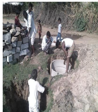
Villagers construct the pits for the IHHL's
