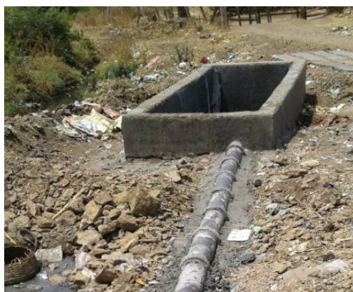
Photos of the Septic tank and connecting pipe near completion - 2017
