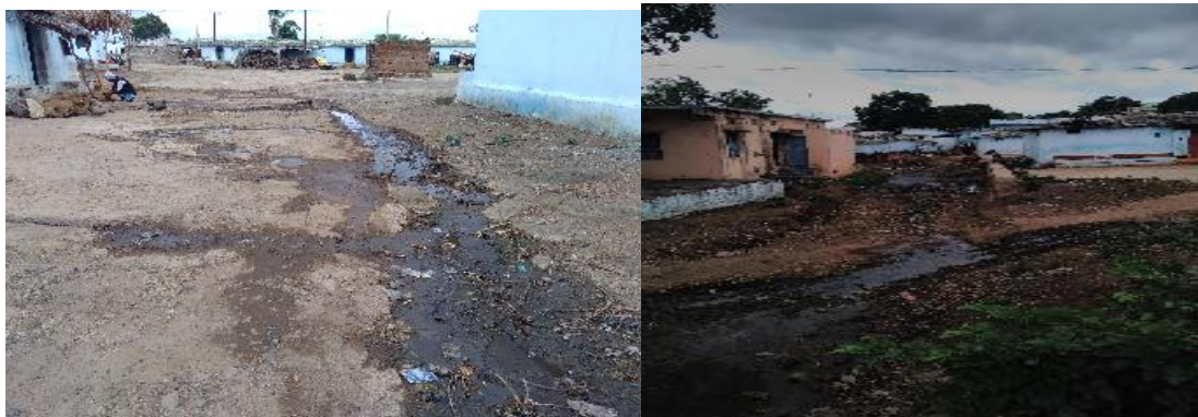
Photos of the existing waste water spilling onto roads – 2013
