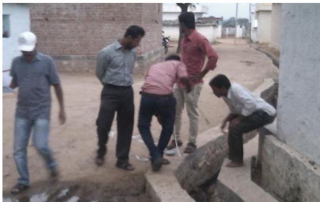
Inspection of the new side drains installed in Sondepur - 2017
