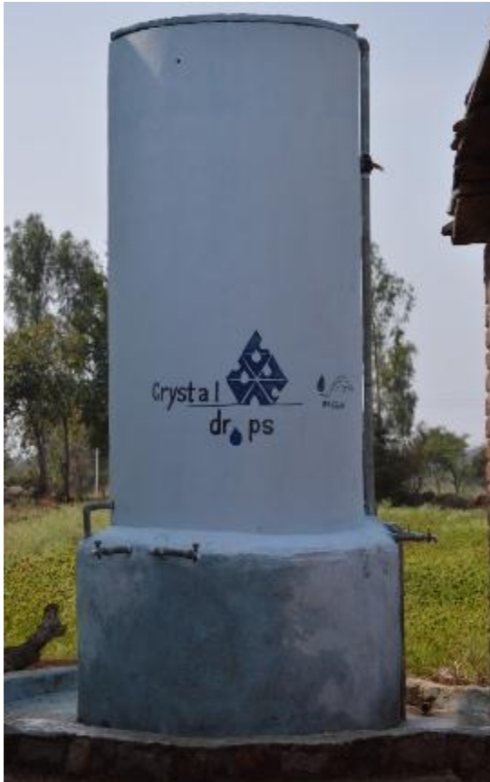
Fully constructed Cistern.
