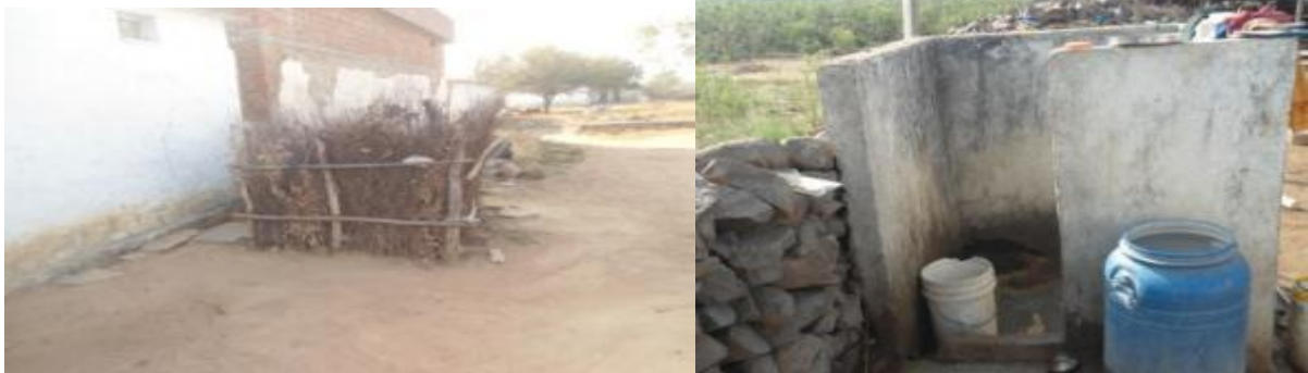
Existing bathing facilities in the villager were minimal – 2013.
